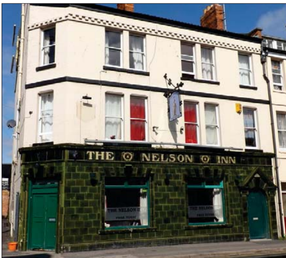
The Nelson Inn, green glazed tiles on the ground floor
