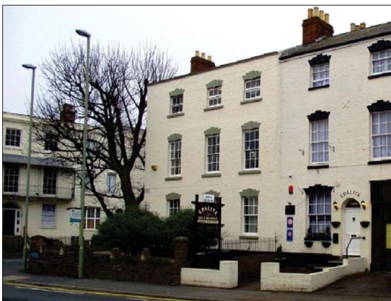
121 Southgate Street beside one of the conservation area's few trees
