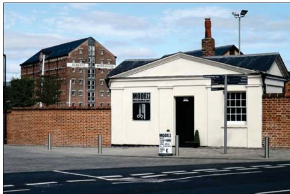
Weighbridge House with dockside warehouses
